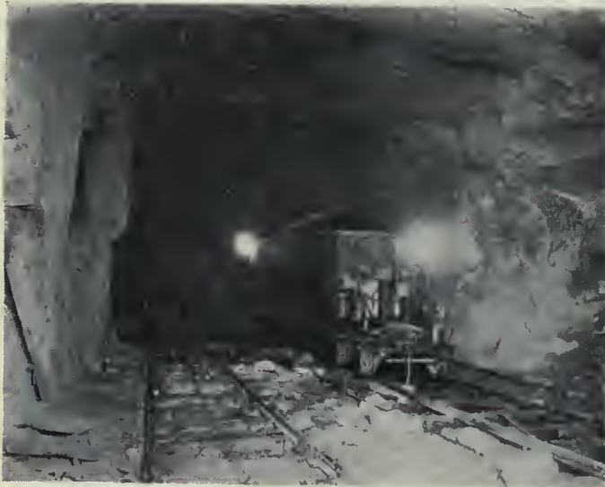
Main Heading Rogers Pass Tunnel—Steam Shovel on standard gauge track at work
